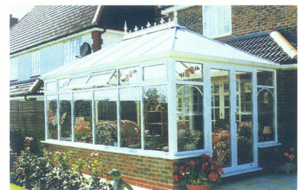
● A typical situation with tiled roof draining onto the box gutter.
